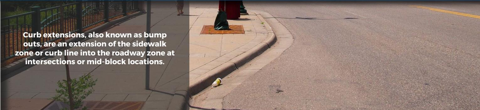
**Curb extensions, also known as bump outs, are an extension of the sidewalk zone or curb line into the roadway zone at intersections or mid-block locations.**
